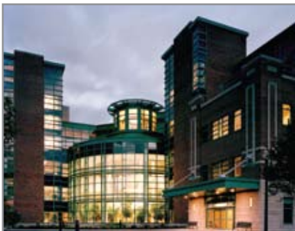
Bronson Methodist Hospital in Kalamazoo, Mich. (photo courtesy Esto Photographics)
